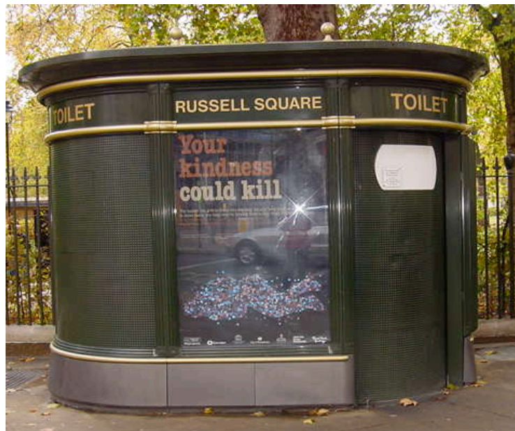
Figure 3. Automatic Public Convenience (APC)
