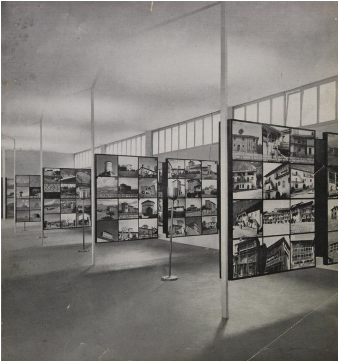
Figure 53. Giuseppe Pagano, Guarniero Daniel, View of exhibition, 'Rural Italian Architecture: Functionality of the Rural House', Milan Triennale, 1936.
