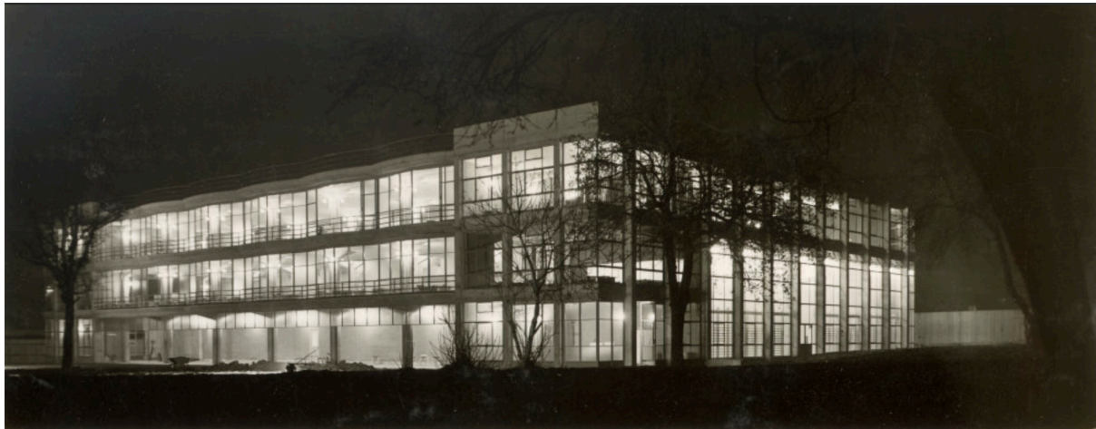
Figure 3 Dell & Wainwright, Pioneer Health Centre, St Mary's Road, Peckham, London, by night, Sir Owen Williams, 1935 , photograph, RIBA7315, RIBA Collections, London.
