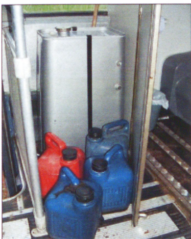
Figure 78: Adapted drinking water tank on board.
