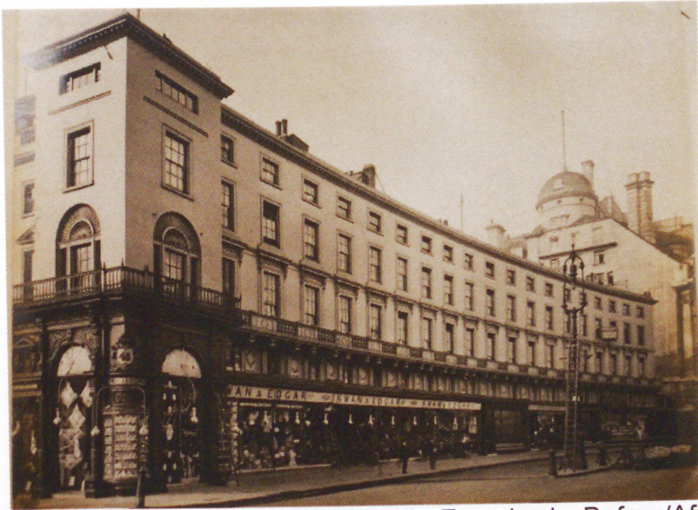
Fig.169 Rebuilding the Quadrant, John Nash's Façade, in Before/After Photographic Survey by John Murray,1940 (CE)
