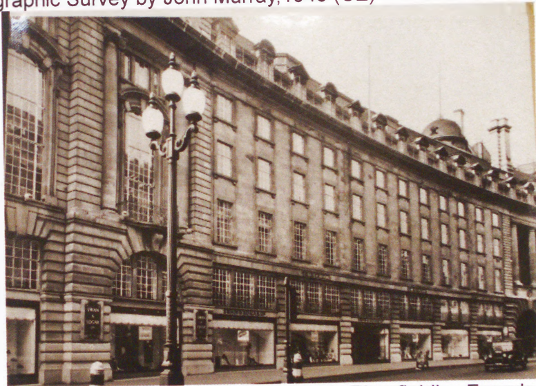
Fig.171 Rebuilding the Quadrant, Reginald Blomfield's Façade, in Before/After Photographic Survey by John Murray,1940 (CE)
