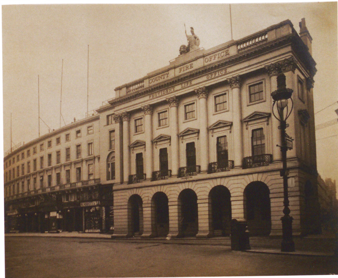
Fig. 130 Nash's façade without the colonnade, in John Murray's photographic survey early twentieth century (CE)
