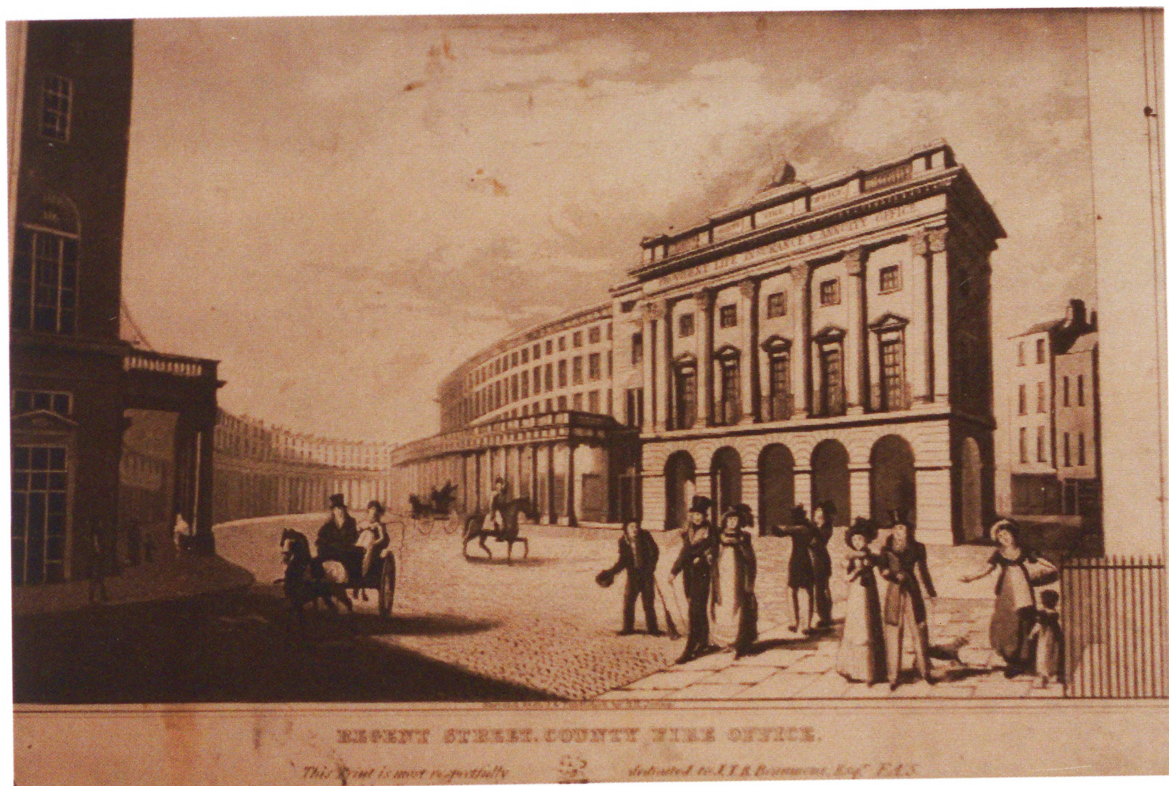
Fig.91 Regent Street, County Fire Office, print by H.Jones (G_MS, Scrapbook relating primarily to the construction of Regent Street, M0017682CL)
