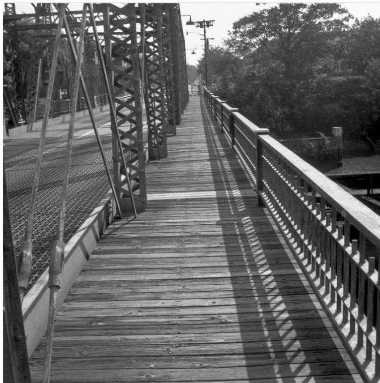
Fig. 26: The Bridge Monument Showing Wooden Sidewalks , as published in: The Monuments of Passaic , Robert Smithson, Artforum (Vol.6, No.4, December 1967), p.49.
