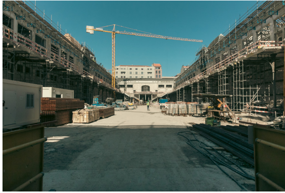
Fig. 98. Mercado do Bolhão renovation site, Porto, Dan Brackenbury, 2019
