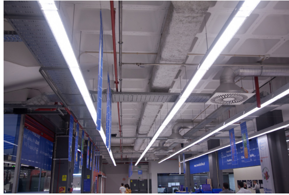
Fig. 103. The bright, fluorescent strip-lighting and bold blue Porto city branding that has been applied uniformly to many of the surfaces in this underground location. Dan Brackenbury, 2019
