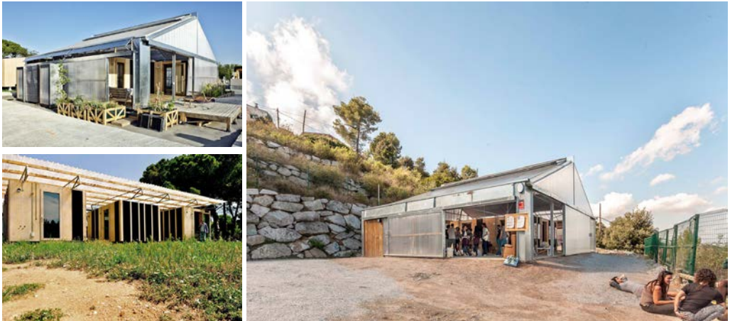
(e)co prototype in three different sites with different layouts: Solar Decathlon Europe competition in 2012 (top left), in ETSAV campus as an educative space (2012-2015) (below left) and in les Planes neighbourhood as a community centre (2015-currently) (right; picture by A. Flajszer).
