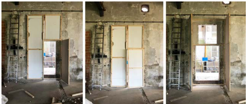
New door connecting new studios with old ones.
