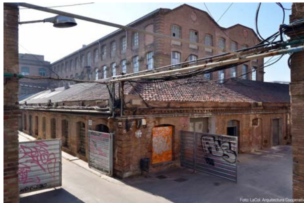
Coopolis warehouse in first term. Behind, the biggest warehouse in Can Batlló, which is planned to become the Barcelona Archive. Source: www.bcn.coop . Image by Lacol.
