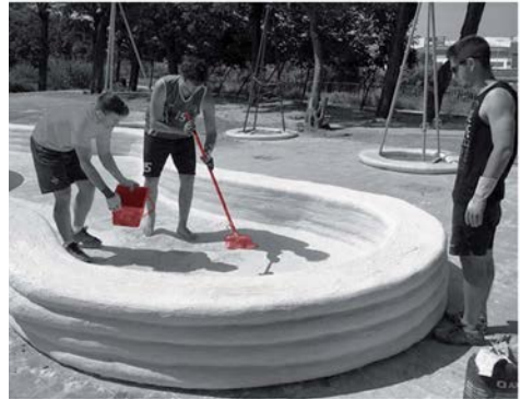
Co-construction workshops of the lavatory using the superadobe building method.
