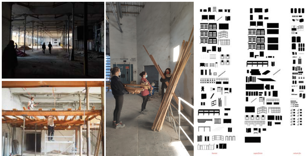
Deconstruction of the mezzanine in Can Batlló warehouses and "harvest map".
