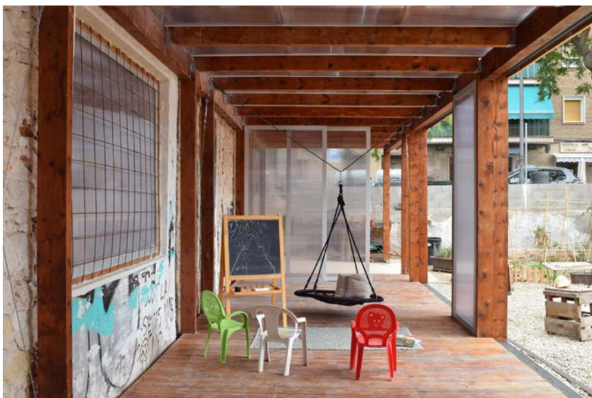
Exterior gallery as built.
