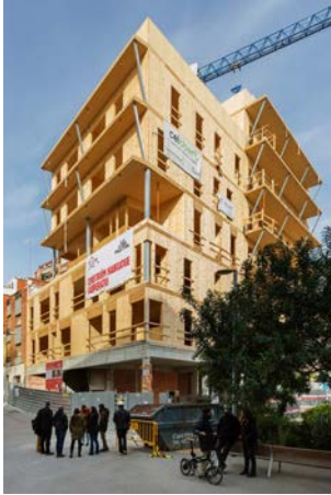
The building under construction with CLT wood.
