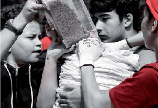
Co-construction workshops of the lavatory using the superadobe building method.
