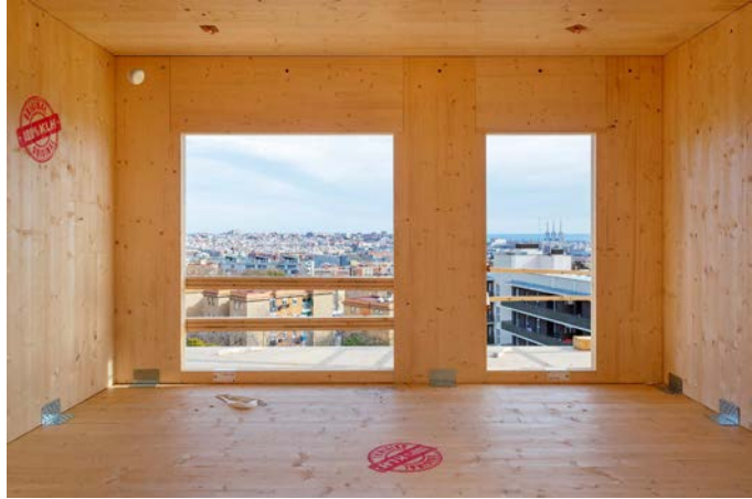
The building under construction with CLT wood.
