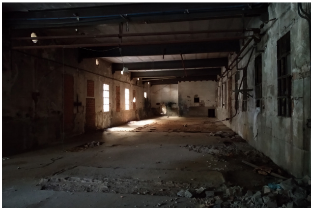
Warehouse L as found.
