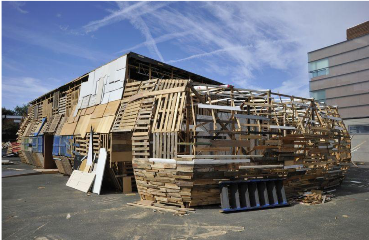
Jellyfish Theater by Kaltwasser and Kobberling, 2010. The first theatre building in London made entirely of recycled materials. The building was used to present a programme of performances about sustainability issues (see Akt II, 2021). Photography by Brian Benson.
