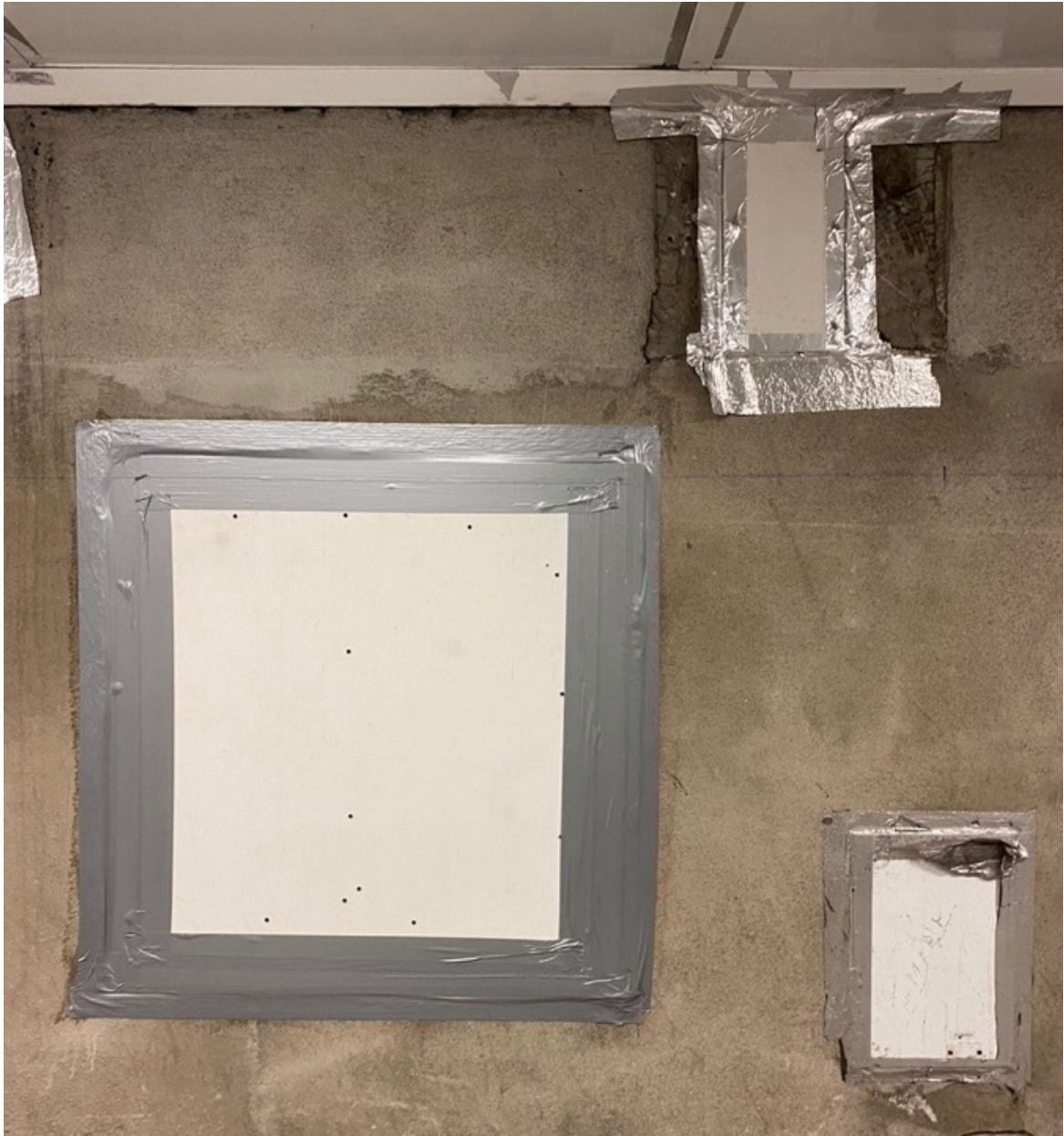
Figure 22. Underground tunnel, London (2020) © 2020 Alison Rees. All Rights Reserved.
