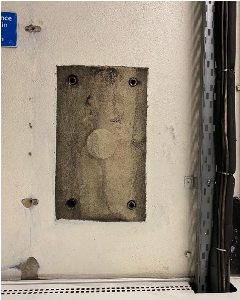
Figure 24. Underground tunnel, London (2020) © 2020 Alison Rees. All Rights Reserved.
