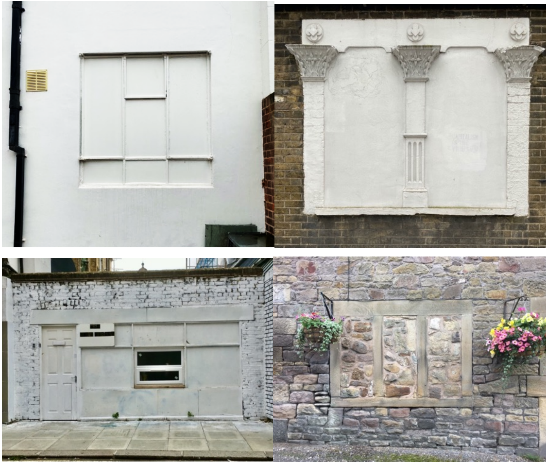
Figure 47. Blocked up windows in various locations, England (2017-2021) © 2017-2021 Alison Rees. All Rights Reserved.
