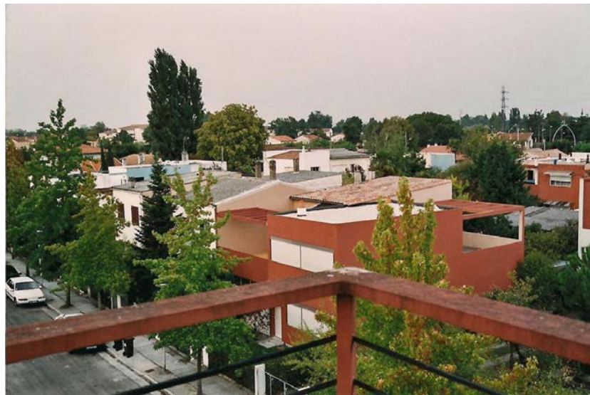
Fig. 8. Cité Frugès's spaces altered by the inhabitants before listing. Here are visible new pitched roofs that enclose the roof garden.
