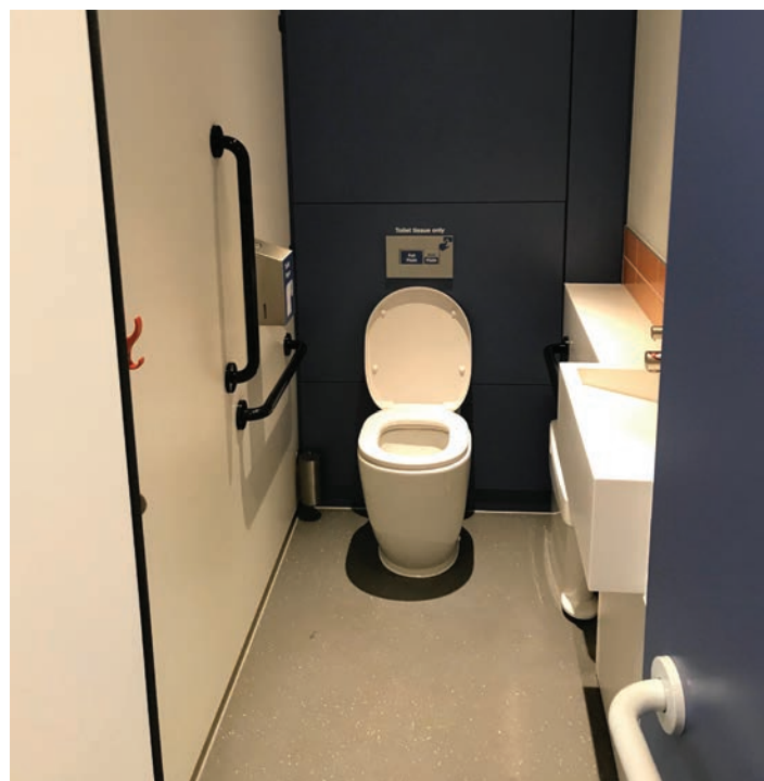
Standard cubicle with hooks, grabrails, single-sheet toilet paper dispenser and shelf; Wellcome Collection. credit: HHCD
