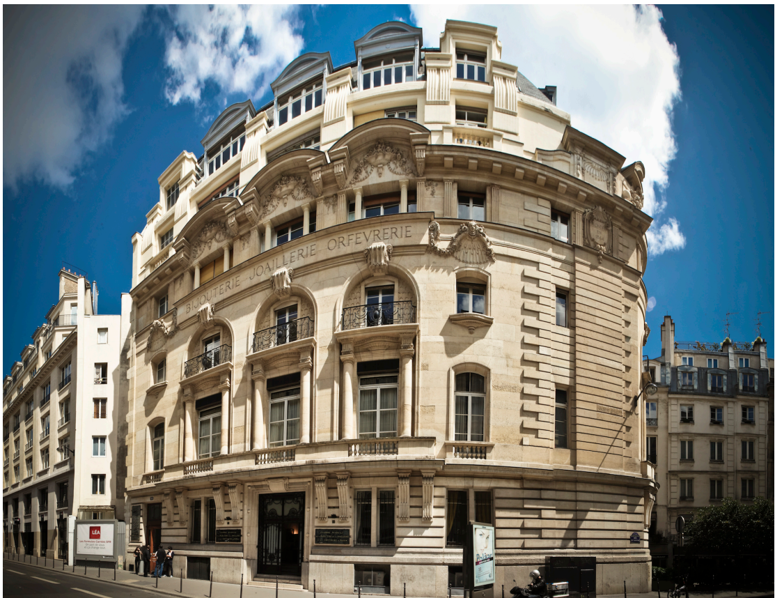
Figure 1: Photograph of the HEJ building at 58 Rue du Louvre, 2019.
