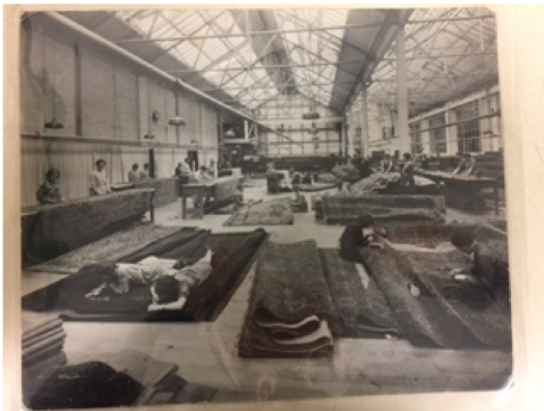
Figure 33: Templeton finishing room, c.1930. (STOD/201/2/15/5/3)
