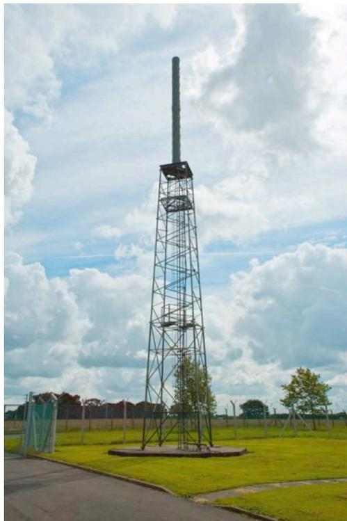
Figure 8.1. Ground-to-air microwave antenna, RAF Neatishead.
