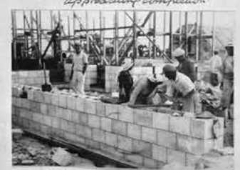
Building the House.
