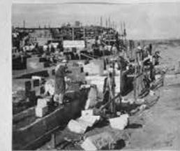
Building the House.
