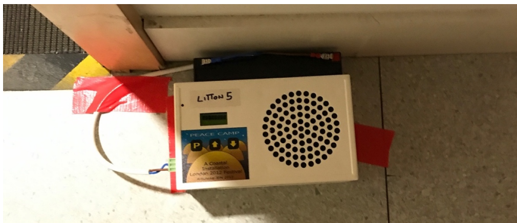
Figure 49. Earcon Loud Speaker, D&D Final Installation
