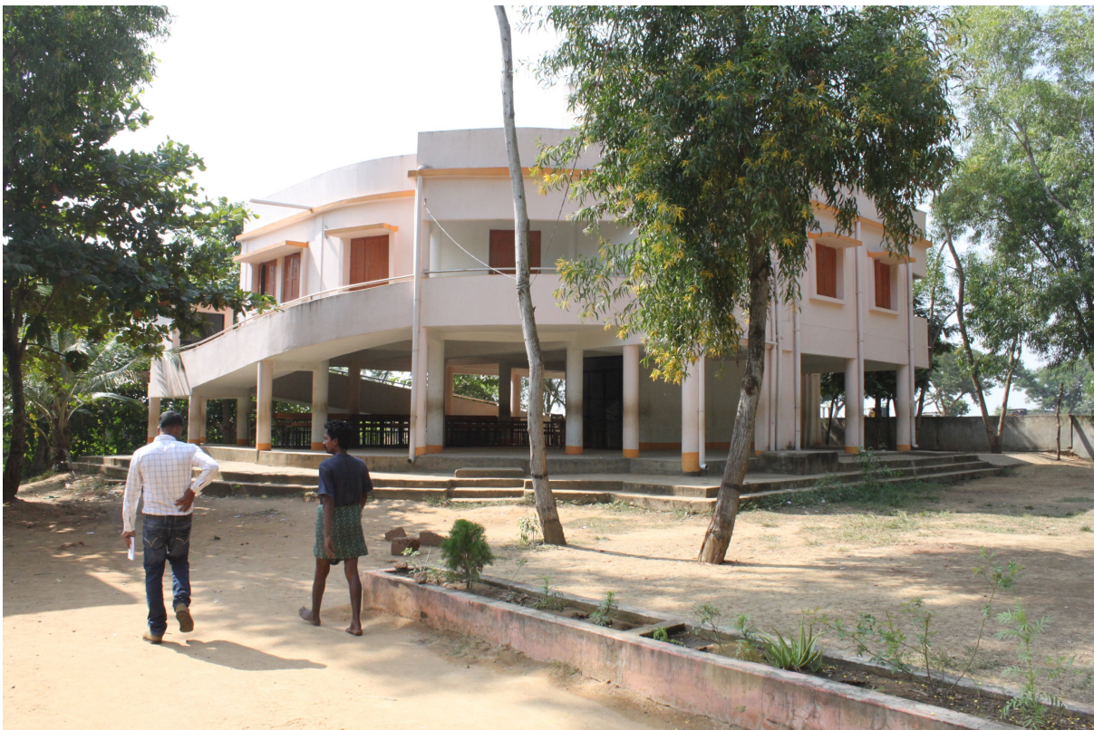
Figure 3.b. Cyclone shelter in Bhubaneswar, India. Photo by Soon Min Hong, 2015.
