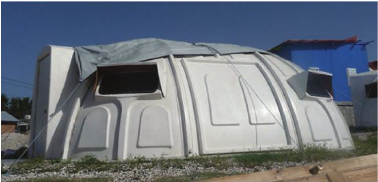
Figure 5. Igloo-style temporary housing in Port-au-Prince, Haiti. Photo by Esther Charlesworth.
