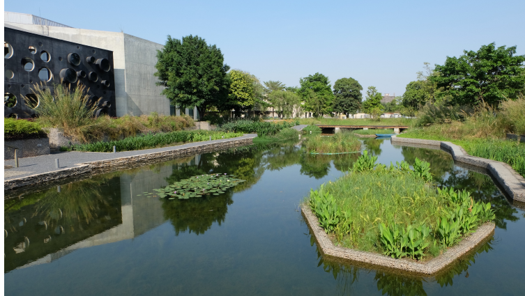
Figure 51: (Left) Foul and rain water filtration beds (photographed by the author)
