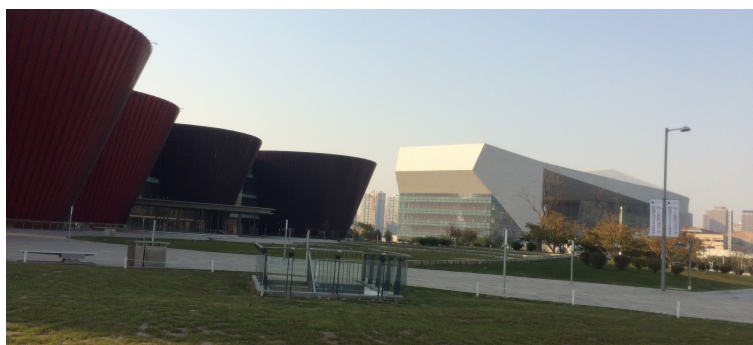
Figure 34: The Shanxi Grand Theatre to the right of the photograph forms the centre piece to the master plan (photographed by the author)
