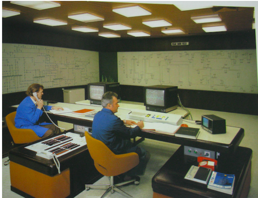
Figure 37. Control station designed by Rade Končar, from Rade Končar, 1946-1986 book, undated
