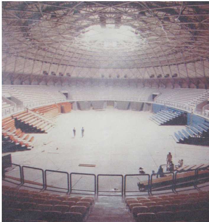
Figure 130. The construction of Cibona Hall, Start , 1987
