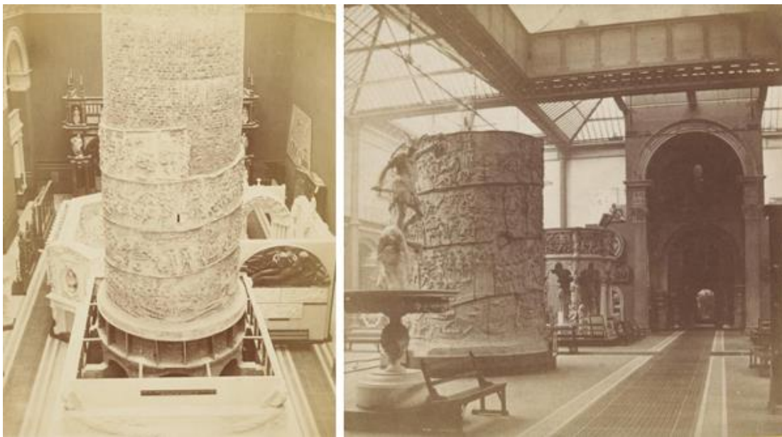
Figure 7.1. The original installation of the reproduction of Trajan's Column around its brick core in the Cast Courts, ca. 1864 © Victoria and Albert Museum, London
