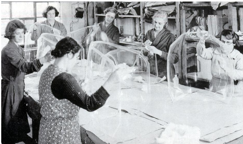
Fig 16. Polishing PMMA cockpit hoods for World War II fighter planes 18
