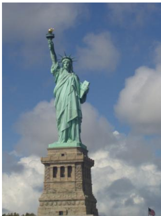
Fig 79. View of the Statue of Liberty, New York, showing a complete green covering of oxidised copper
