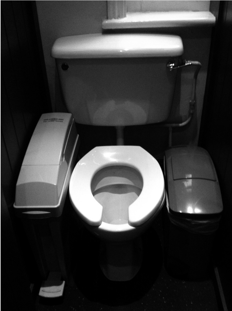
Figure 7. Multiple sanitary bins in standard cubicle illustrate the failure of the infrastructure to consider menstruation. In addition, a lack of consideration in the servicing of bins presents a further compromise of space. (Source: Bichard, 2011)
