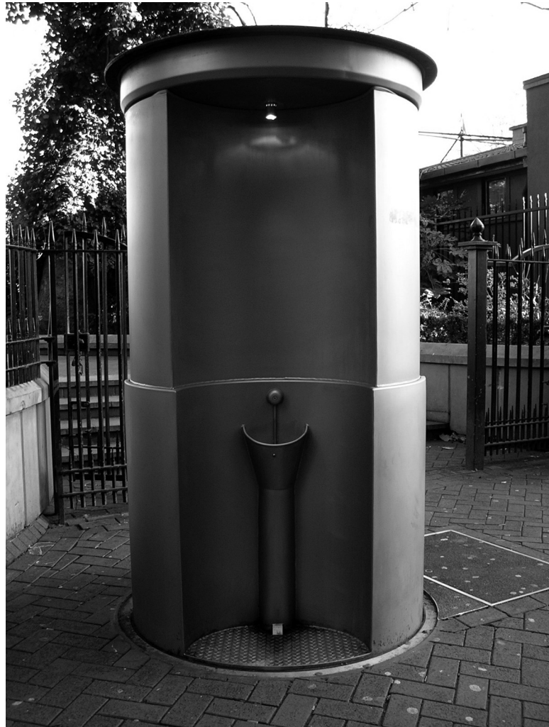
Figure 6. Permanent retractable urinal that comes up at dusk and goes down at dawn. (Source: Bichard, 2005)
