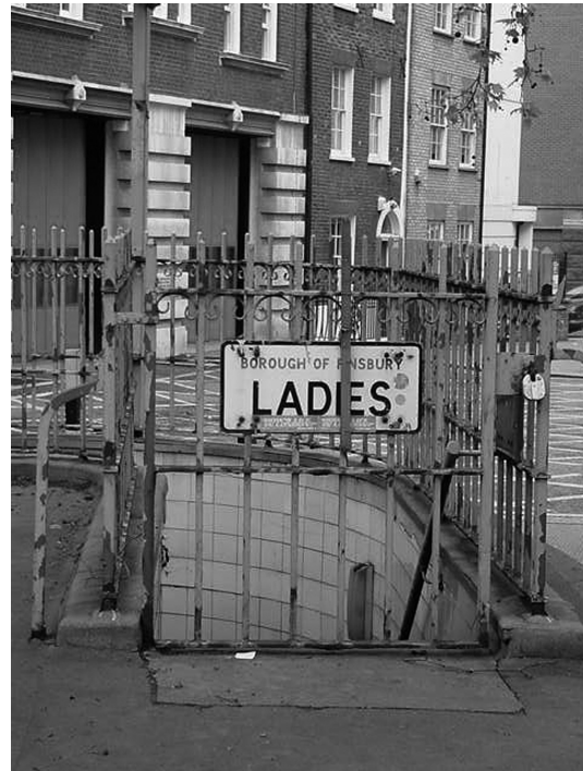
Figure 2. Ladies Victorian subterranean toilet in Clerkenwell, London. (Source: Bichard, 2004)
