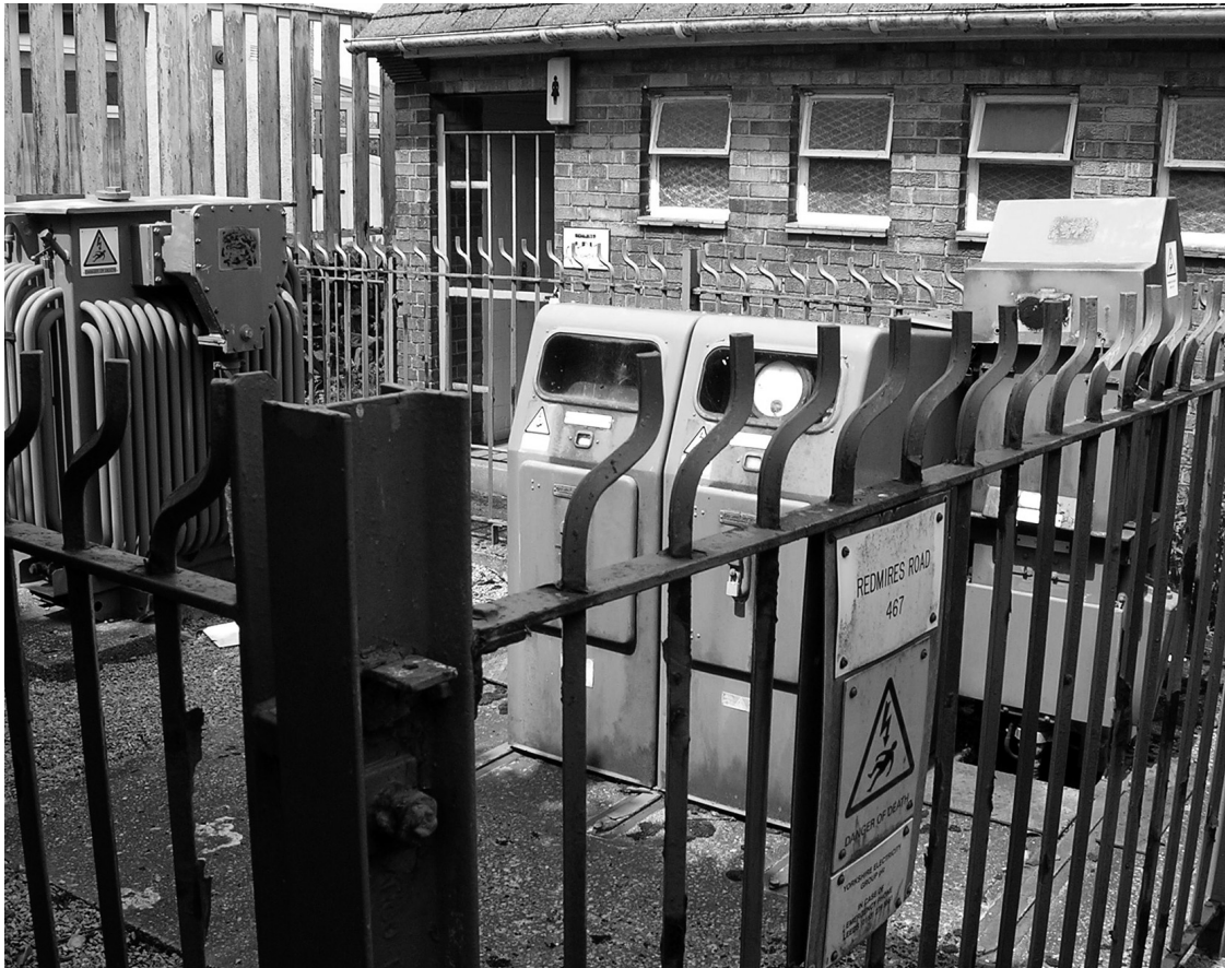
Figure 12. Toilets with poor natural surveillance can be intimidating. This block is located behind an electricity ‘sub station’. (Source: Bichard, 2006)
