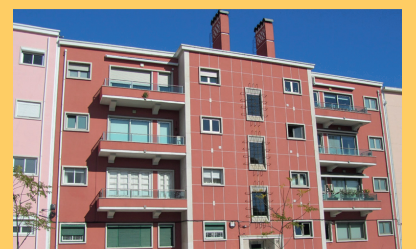
Building in Cell IV
