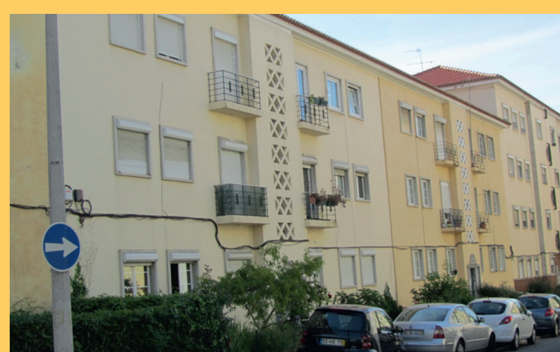
Building in Cell I
