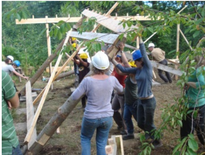
Students studying at CAT erect a timber structure
