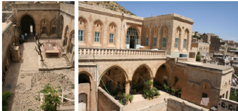
Figure 7: Thresholds in the building configuration. Photographs: Author.
