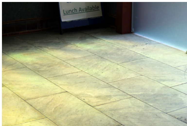
Site 3, vestibule floor. Photograph: Author
