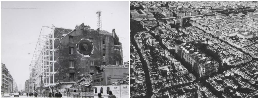
Fig. 53 (left) Gordon Matta-Clark, Conical Intersect , 1975; (right) View of the completed Centre Pompidou, 1977.
