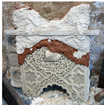
Figure 1.05: The drawn, drypoint design and carving plasterwork [Photo: Owen Johnson]
