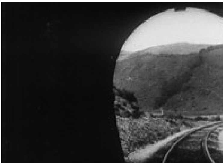
Figure 26: The Haverstraw Tunnel (1887) The Biograph Company
