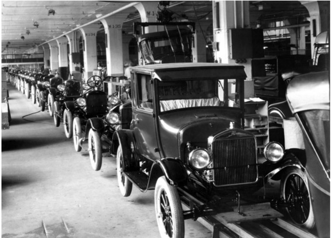
Figure 36: Ford Model T production line.
