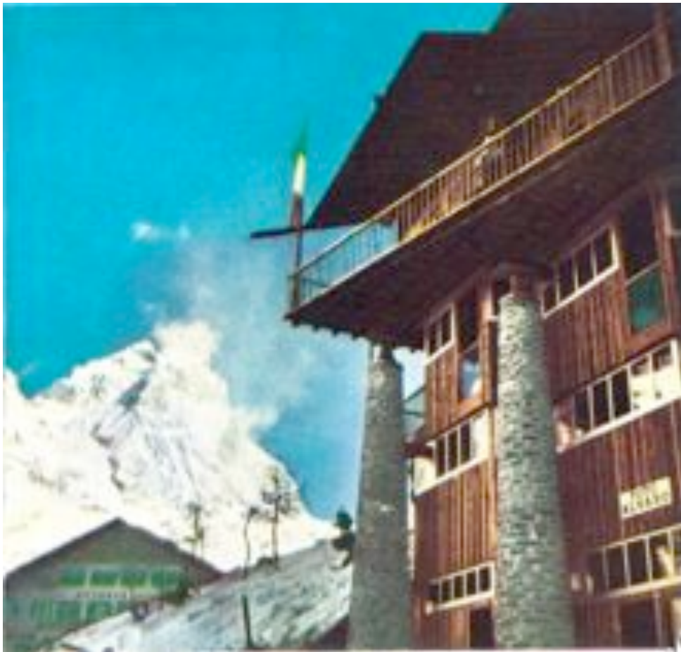
Illustration 47. Rifugio Ragazzi Pirovano , youth hostel designed by Franco Albini in Cervinia, in the Valle d'Aosta, Italy, 1948 – 1952.
