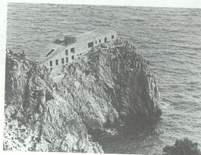
The building site of Casa Malaparte, Capri, 1940
